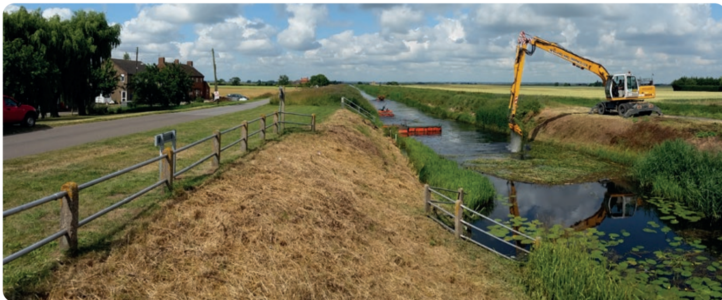
Maintenance work by Welland and Deepings Internal Drainage Board
